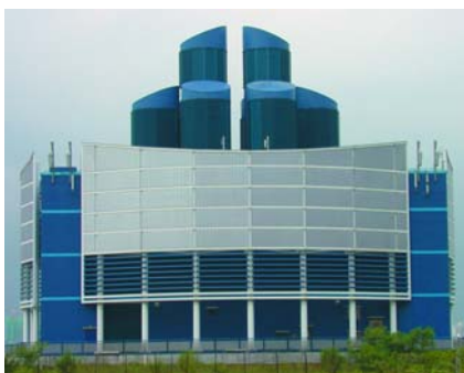
Western Harbour Tunnel, Hong Kong. Triple bank faceted circular louvre installed to handle the high air volumes required and to provide maximum rain protection even in typhoon conditions.
