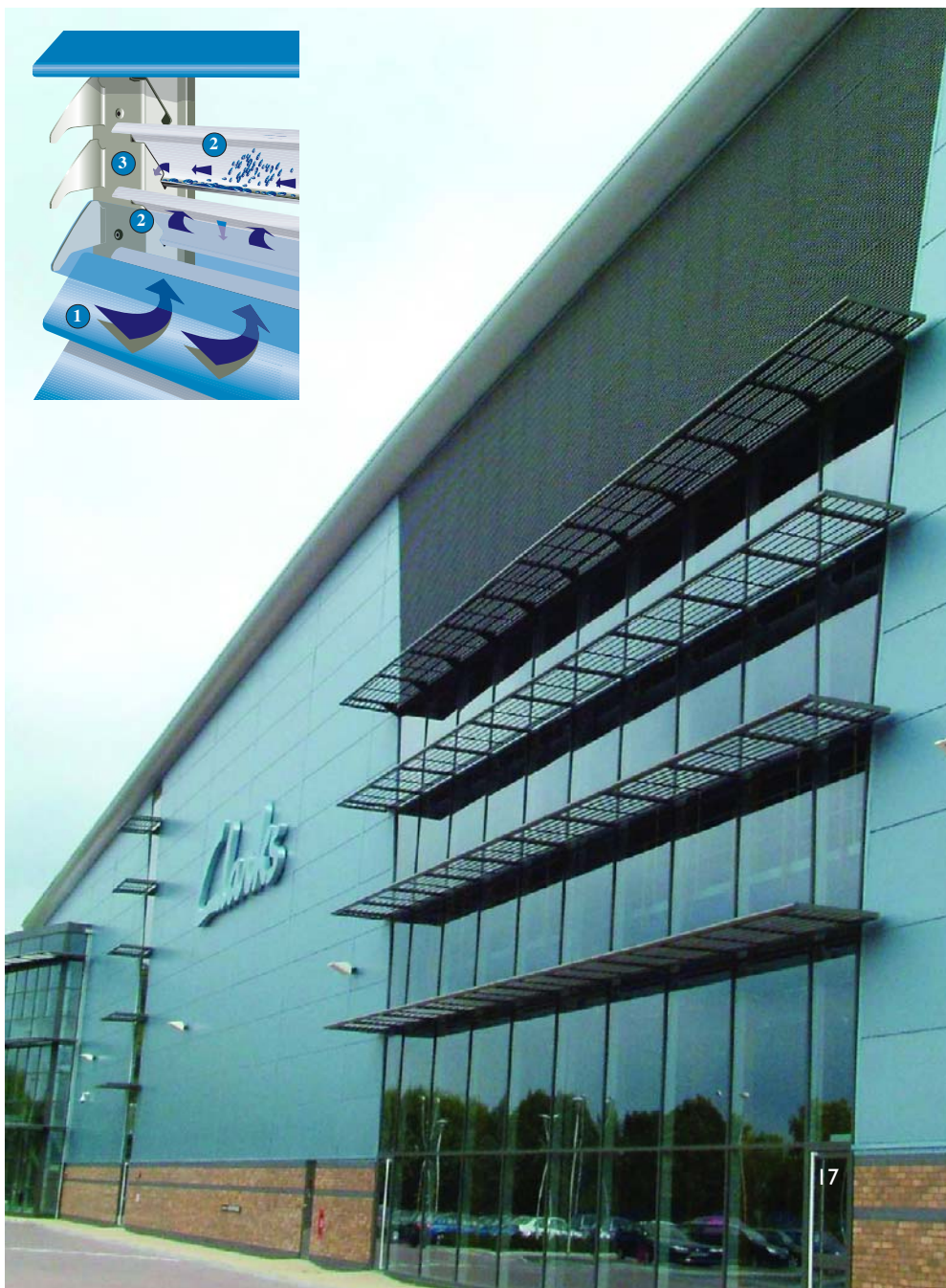
Clarks Shoes, Somerset. Universal Louvre for screening in both painted and pre-coated finishes.
