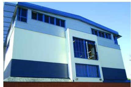
Crawley College, Crawley. ERD louvre panels on the plant room, and Solarfin solar shading panels.
