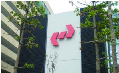
Kowloon Canton Railway Corporation, Hong Kong. Colt inverted Universal Louvre is used extensively for this new underground station to provide high volume airflow with rain defence for plant rooms, entrances, vent shafts and external decoration.
