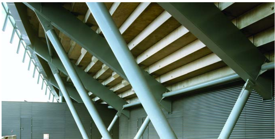
ERD rain defence louvre to plantroom enclosures.
