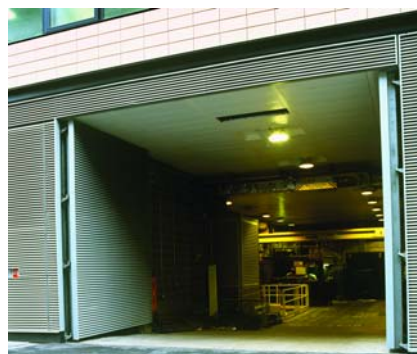
UCL, London. Louvre doors to loading bay.
