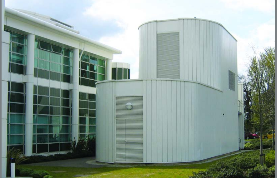
National Physical Laboratory, Teddington. 1ULISH panels with upgradeable 2ULISH panel sections.
