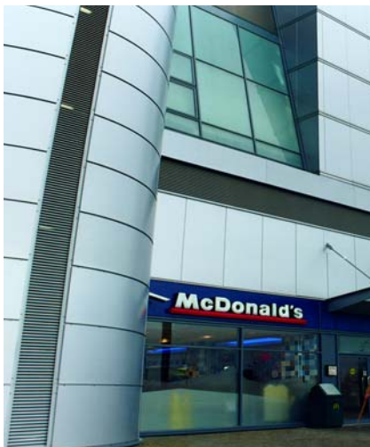
Xscape, Milton Keynes, UK. 2000m 2 of Universal Louvre including both Colt Single Bank and Double Bank Universal rain defence louvre.
